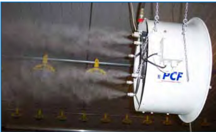
Figure 113: Example of spray cooling system.
