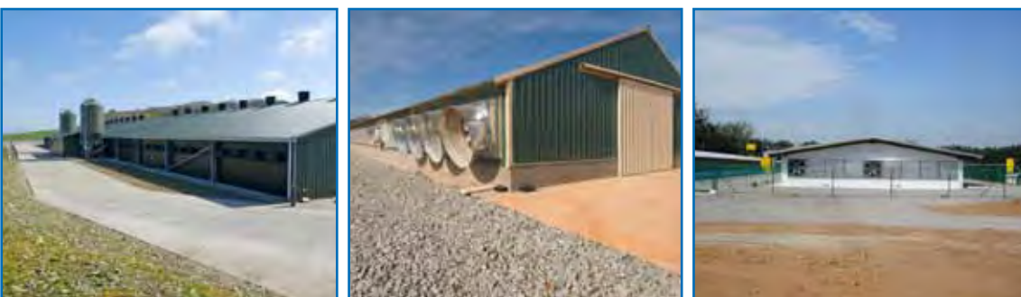
Figure 6: Houses with a low biosecurity risk showing concrete areas and no vegetation around perimeter of the house.
