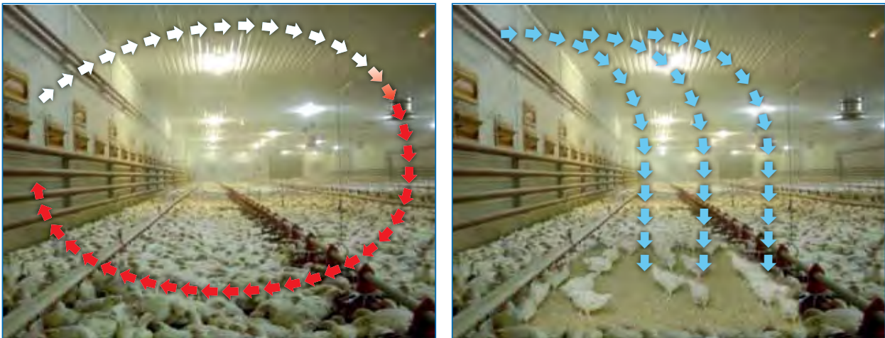
Figure 108: Illustration of airflow into the house. The picture on left shows a correct fast airflow during minimum ventilation, the picture on right shows an incorrect slow airflow during minimum ventilation.
