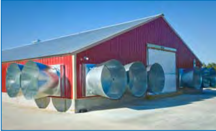
Figure 110: Example of a typical tunnel ventilated house.
