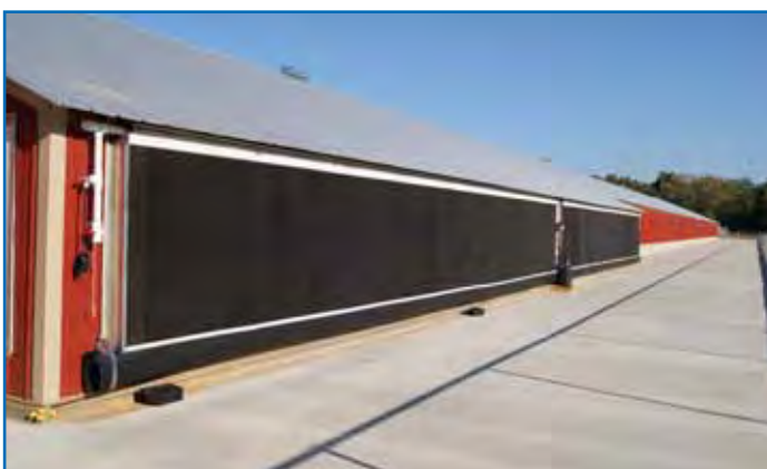
Figure 114: Example of a cooling pad.
