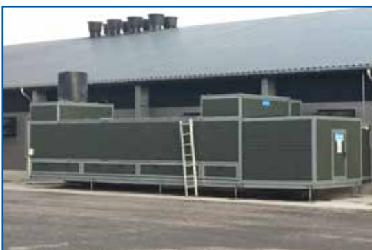
Figure 2.6: Example of a heat exchanger.
