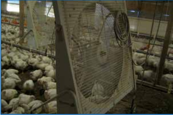
Figure 6.2: Circulation fans in a naturally ventilated house.
