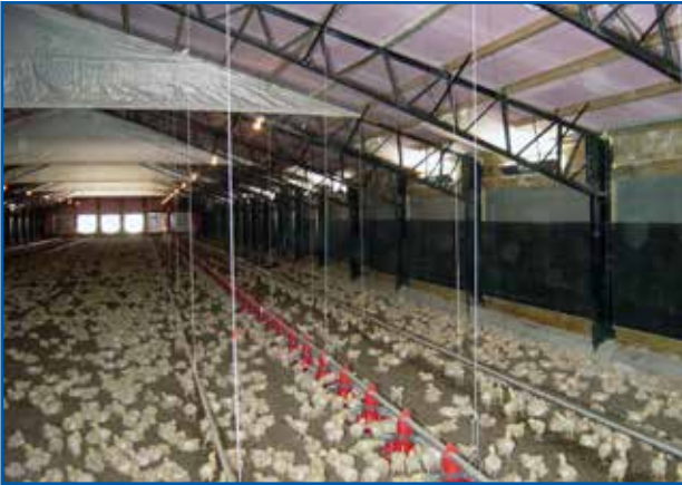
Figure 6.10: Internal view of house in transitional ventilation mode. Inlets are fully opened and the tunnel fans are running. Bird distribution shows birds are comfortable.
